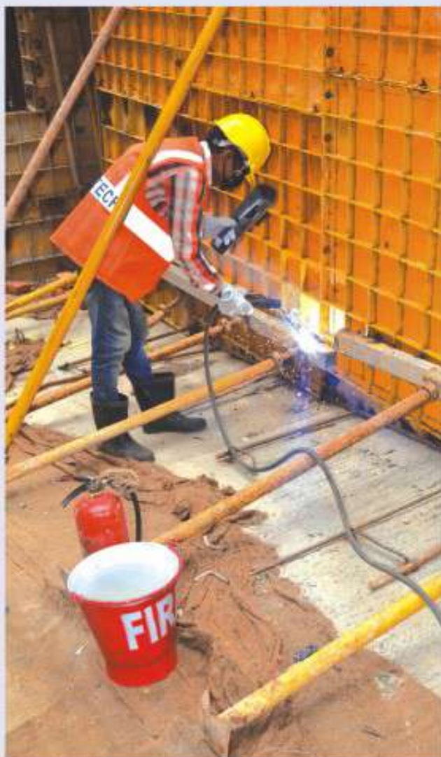
PPE (helmet, welding hand screen, hand gloves, gum boot and safety vest) worn by worker while welding at Sheltech Astra
