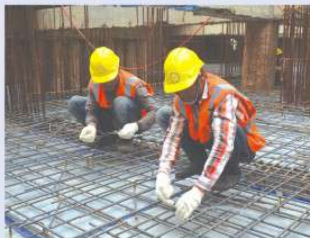
PPE (helmet, hand gloves, gum boot and safety vest) worn by workers while fabricating reinforcement at Sheltech Astra
